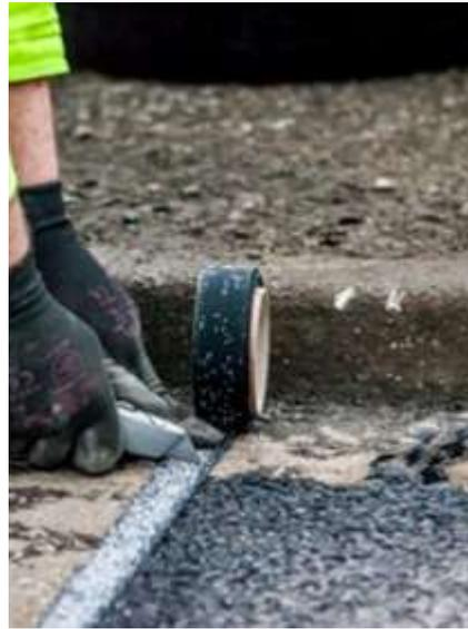
Remove product from its packaging, roll out on to the road surface, beaded side up. Heat the material until it starts to bubble and melt.
