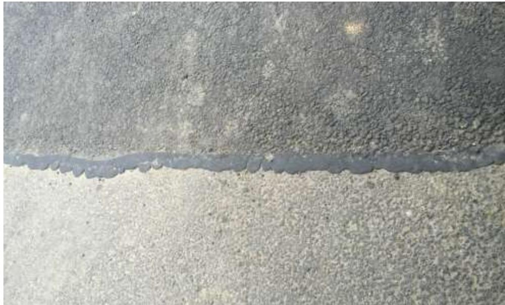
Sealing the joints of a repair to prevent water ingress and progressive fretting makes sense.
